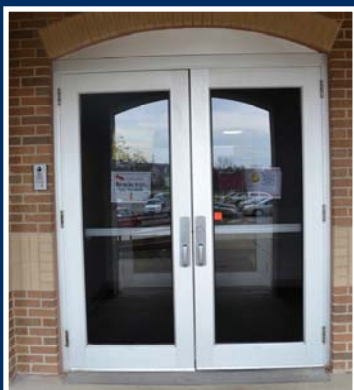
New door buzzer system at Heritage MS
