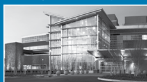
Dublin Methodist Hospital
